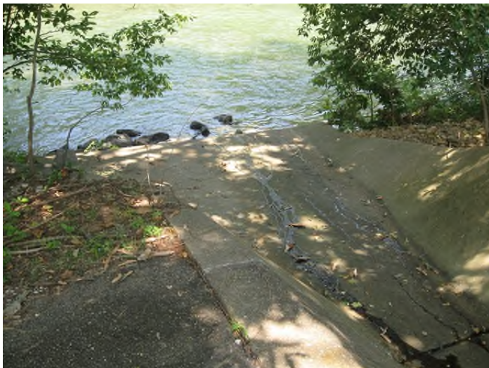
Concrete channel at river
