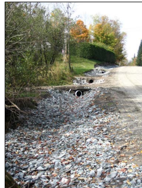
18" culverts (driveway culverts may be 15")
