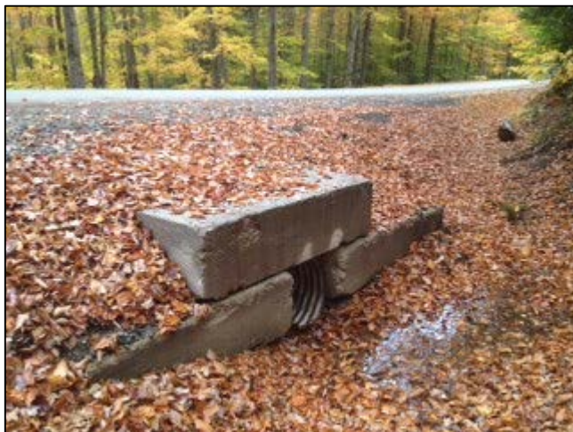
Culvert end treatments
