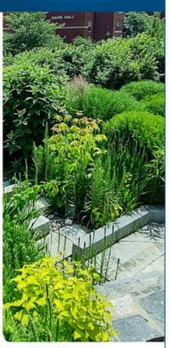
Bioretention Basin at Providence College Image: Rhode Island Stormwater Innovation Center
